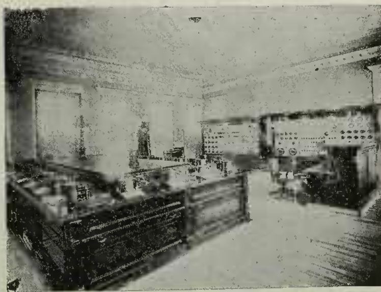
Força Policial — Sala dosapparehos no Quartel principal
